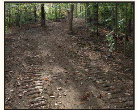
Figure 2: A skid road used to safely transport timber logs while minimizing compaction to surrounding forest
