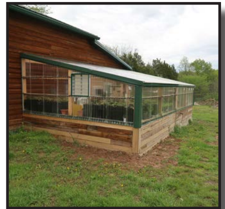
Photo 3: The completed greenhouse.
