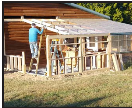
Photo 2: Greenhouse addition under construction.
